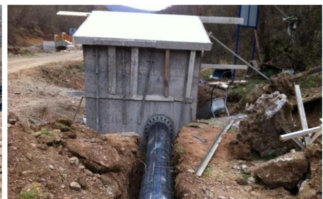
Figure 14: Open channels with excavators and connecting penstock with hydropower house
